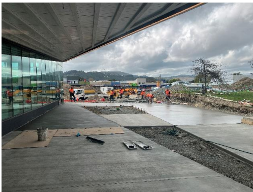
Concrete civil works progressing outside the Community Room.
