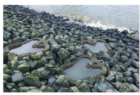
Figure 1.25 Tide pools installed in rock revetment. Ref SHRP
