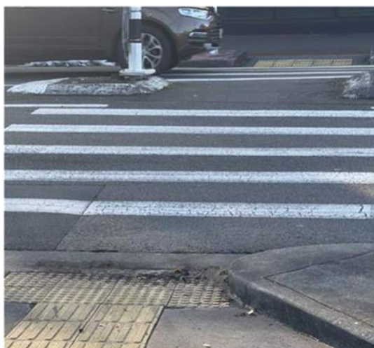
Figure 4: Tactile pavers conflicting with vertical kerb at Bloomfield Terrace
