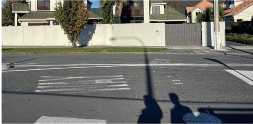
Figure 13: Ghost markings at Hautana Street
