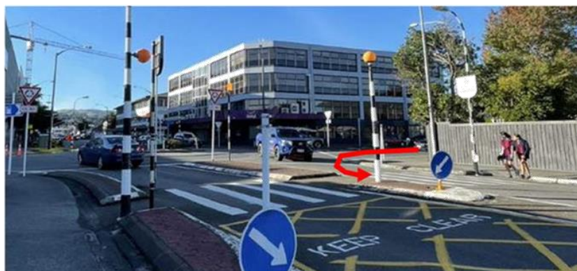
Figure 8: Pedestrian crossing hidden on the southern approach
