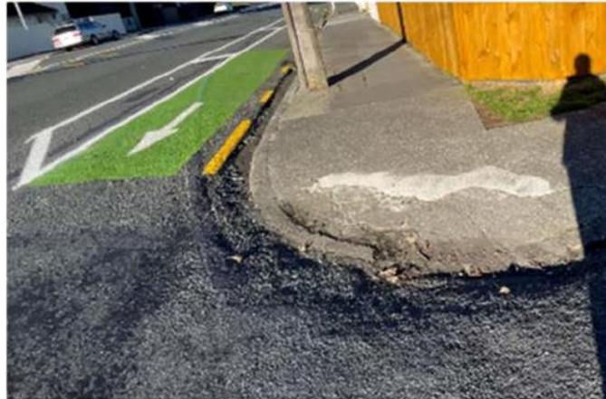
Figure 2-7 Pedestrian kerb ramp on the eastern side of Willoughby Street
