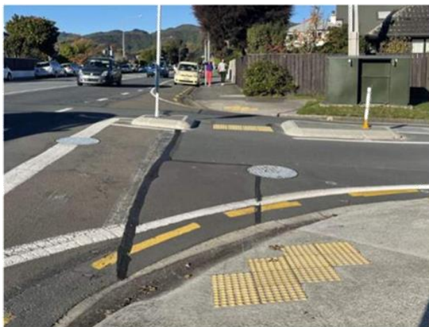
Figure 5: Smooth pedestrian ramps and tactile pavers at Colin Grove
