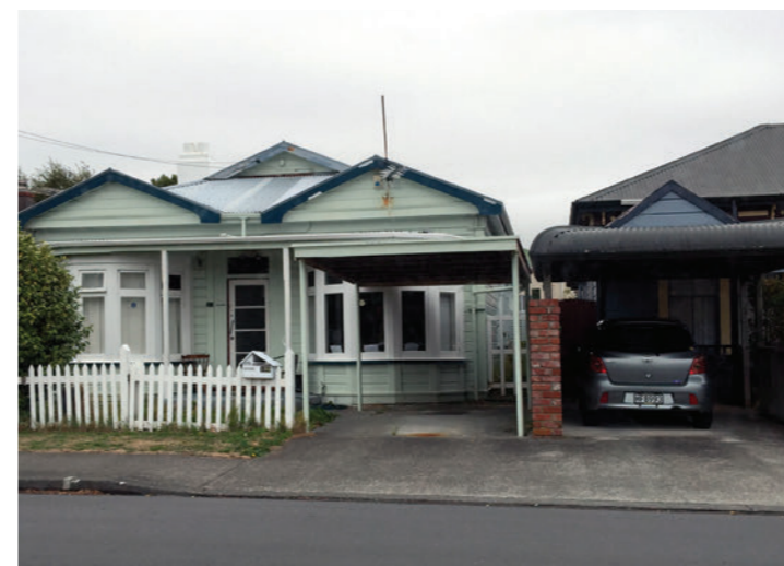
Some eroding of front yards with off street parking compromising the quality of the housing.
