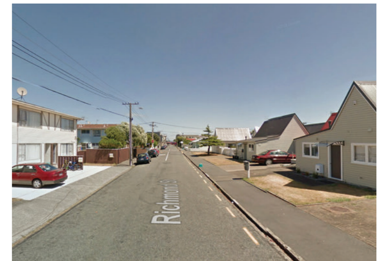
Richmond St multi-unit redevelopment of low quality housing that does not support local character.
