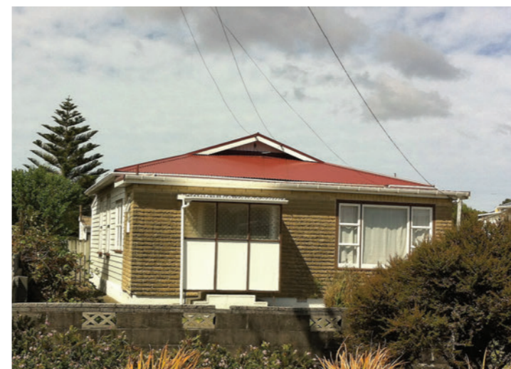
Unsympathetic alterations erode local character.
