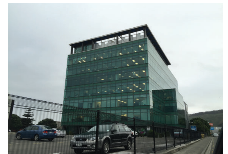
Occasional larger scale office buildings surrounded by empty car parking areas with no positive landscape quality
