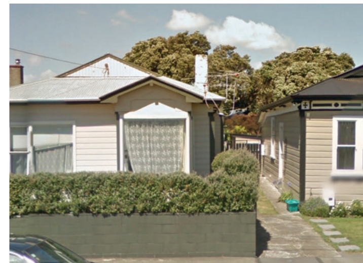
Unsympathetic modifications with loss of original architectural detail.
