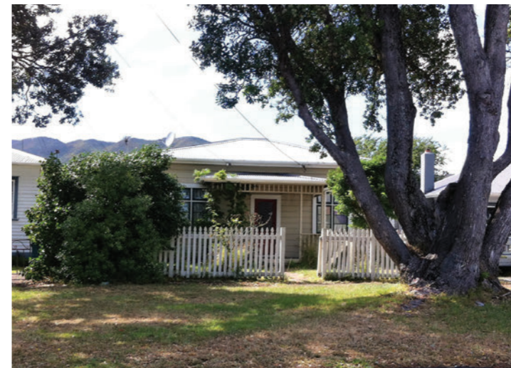
Traditional period housing (early 1900s) within a mature tree streetscape.
