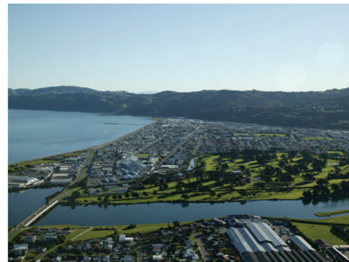
Hutt River Corridor
