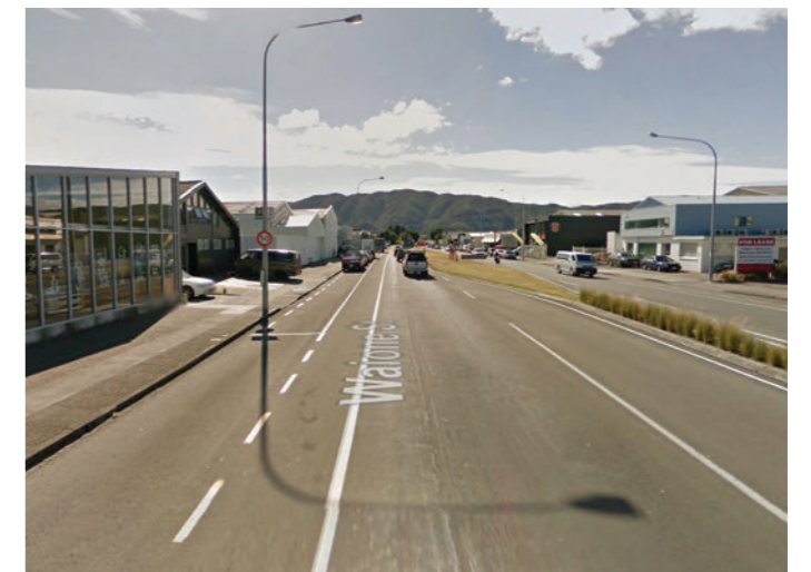
Commercial character (Waione Street)
