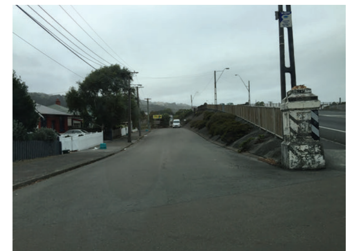
Poor connection over rail lines to Alicetown
