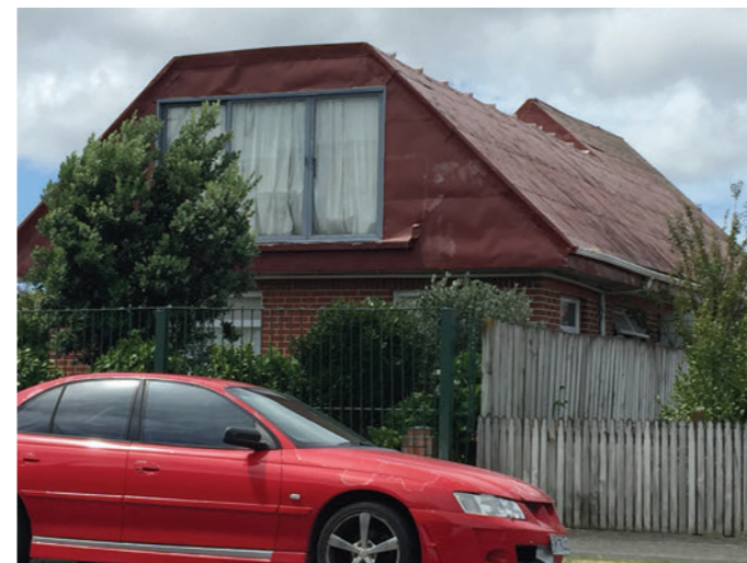
Variable quality of Cuba Street building stock
