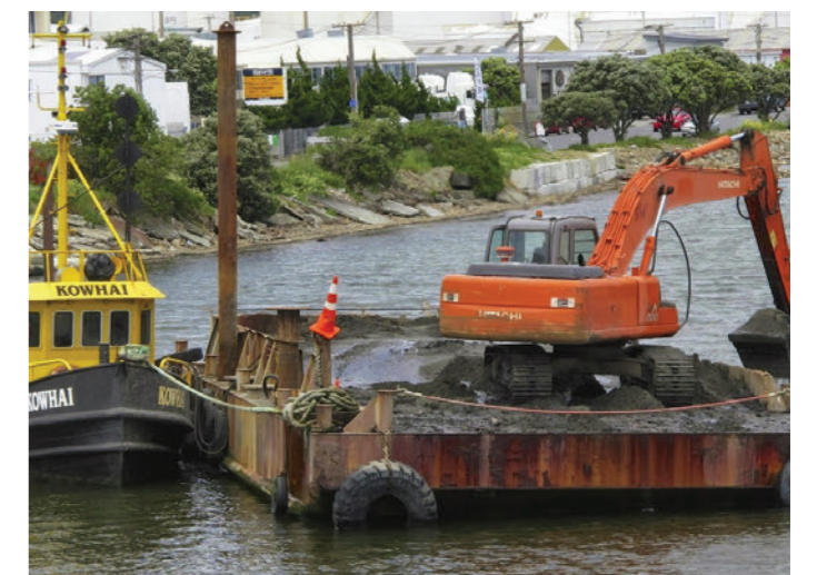
Dredging operation on Hikoikoi reserve
